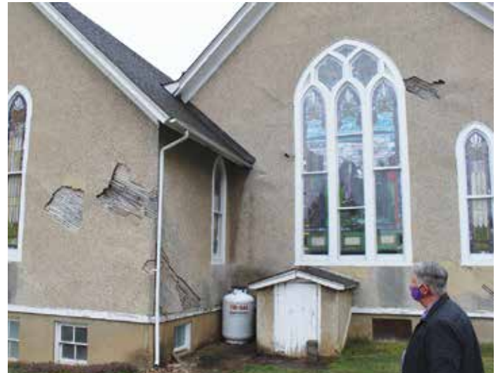
Dick Story, Chair of the Fundraising Committee, and parishioner of the church, points to the large holes on the original siding.
